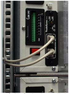
Parallel configuration and programmable relay contacts board
